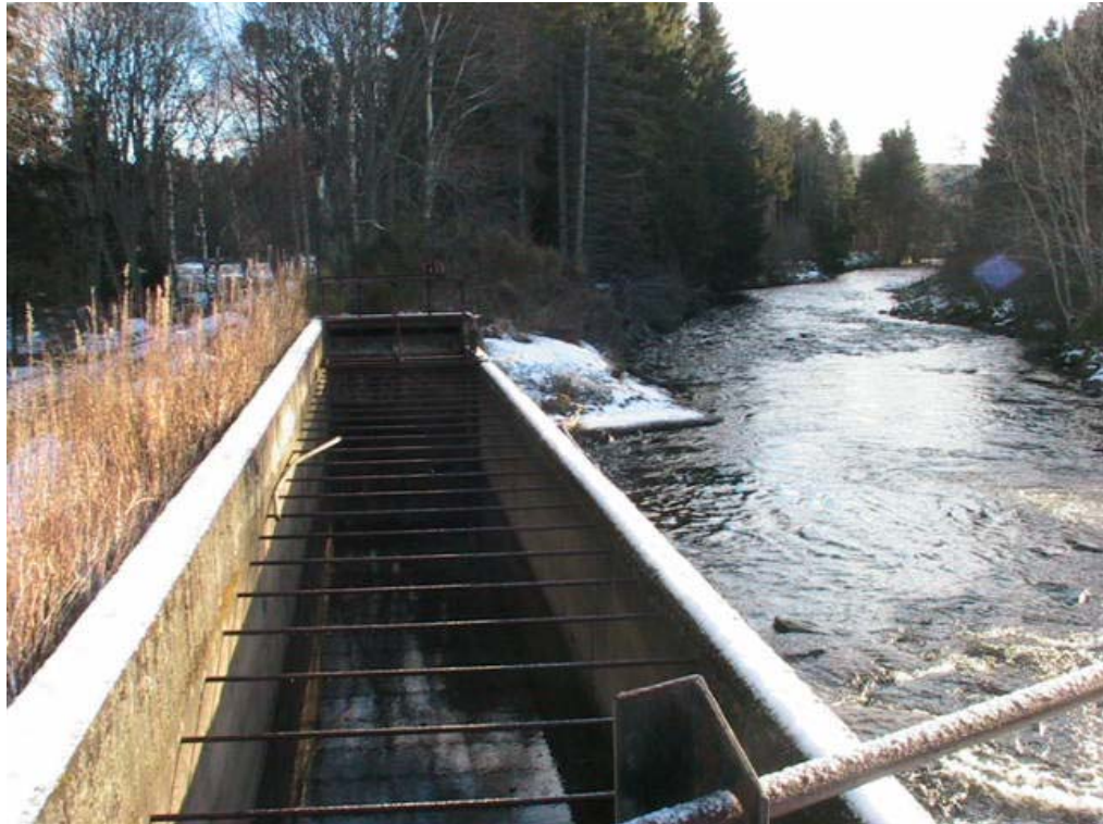
Fig. 3. Existing intake, looking downstream
