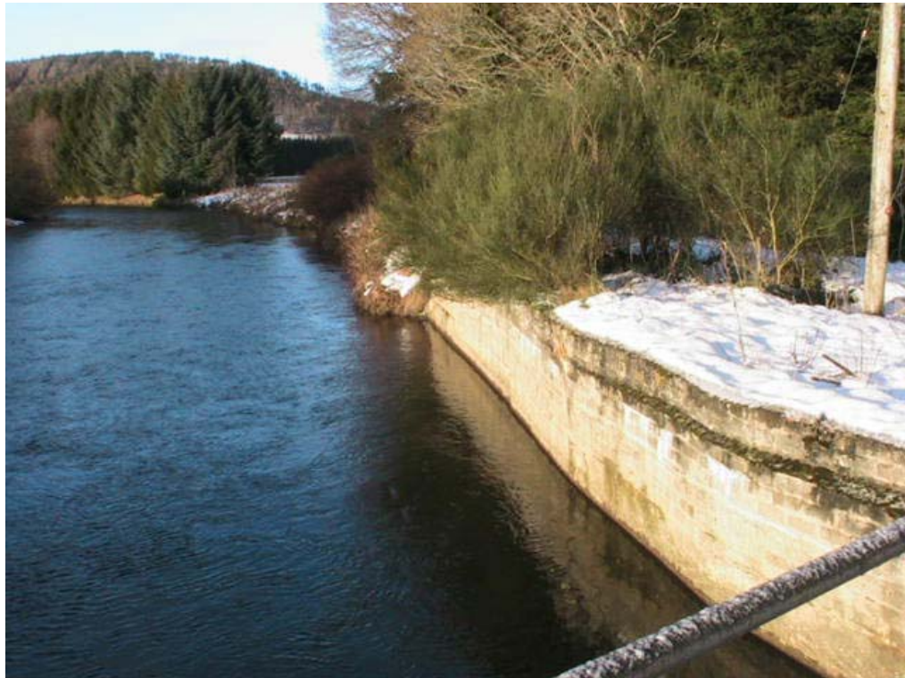
Fig. 5. Looking upstream, position of new intake in existing wall
